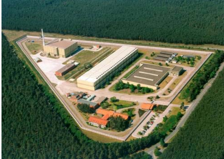
Figure D–1: Interim storage facilities and pilot conditioning plant at the Gorleben site (Copyright: BLG)
